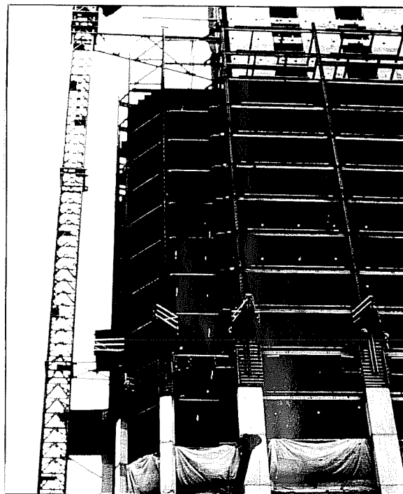
Fig. 1.1b Forty-nine Story First City Tower, Houston 2 (Courtesy of Walter P. Moore & Associates)
